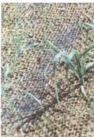
WHEN WOVEN, AS ABOVE, COCONUT HUSK TWINE ACTS AS A NATURAL EROSION CONTROL OPTION, SHOWN HERE.
